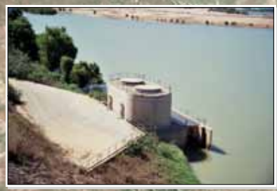
TOM FENWICK No.4 & 5 PUMP STATION
