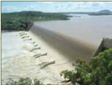
BURDEKIN FALLS DAM - Capacity 1,860,000 Megalitres
