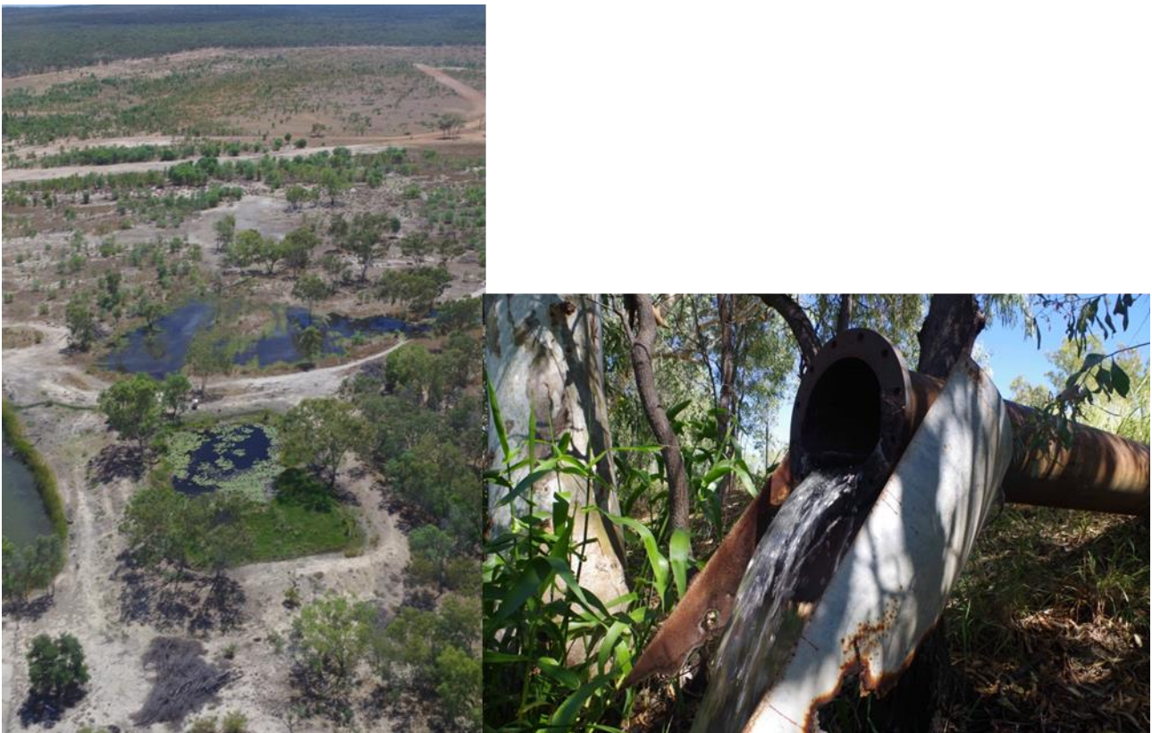
Figure 2. Joshua spring enclosed within a rectangular shaped 'turkey nest' in the foreground (left); the outflow pipe (right) is through the right-hand wall.
