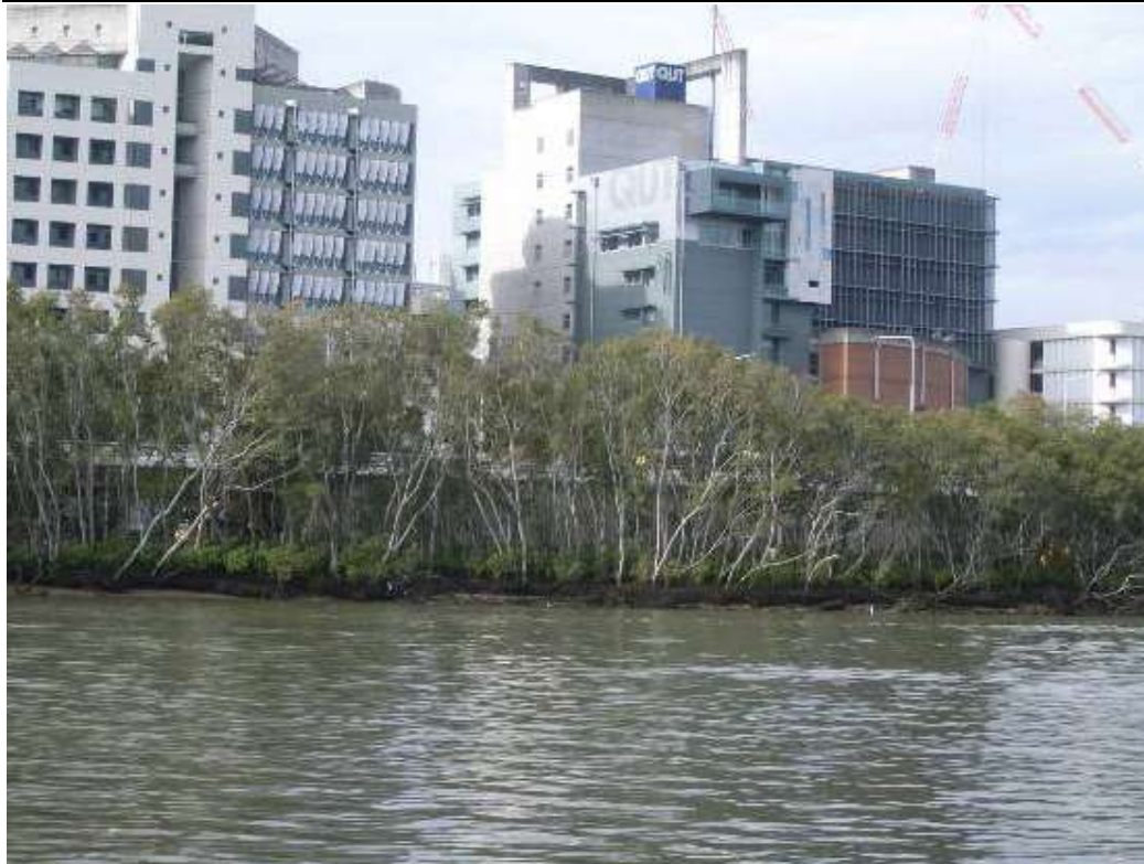
Photograph 2 Eroded mangroves adjacent to QUT and Riverside Expressway, South Brisbane Reach.
