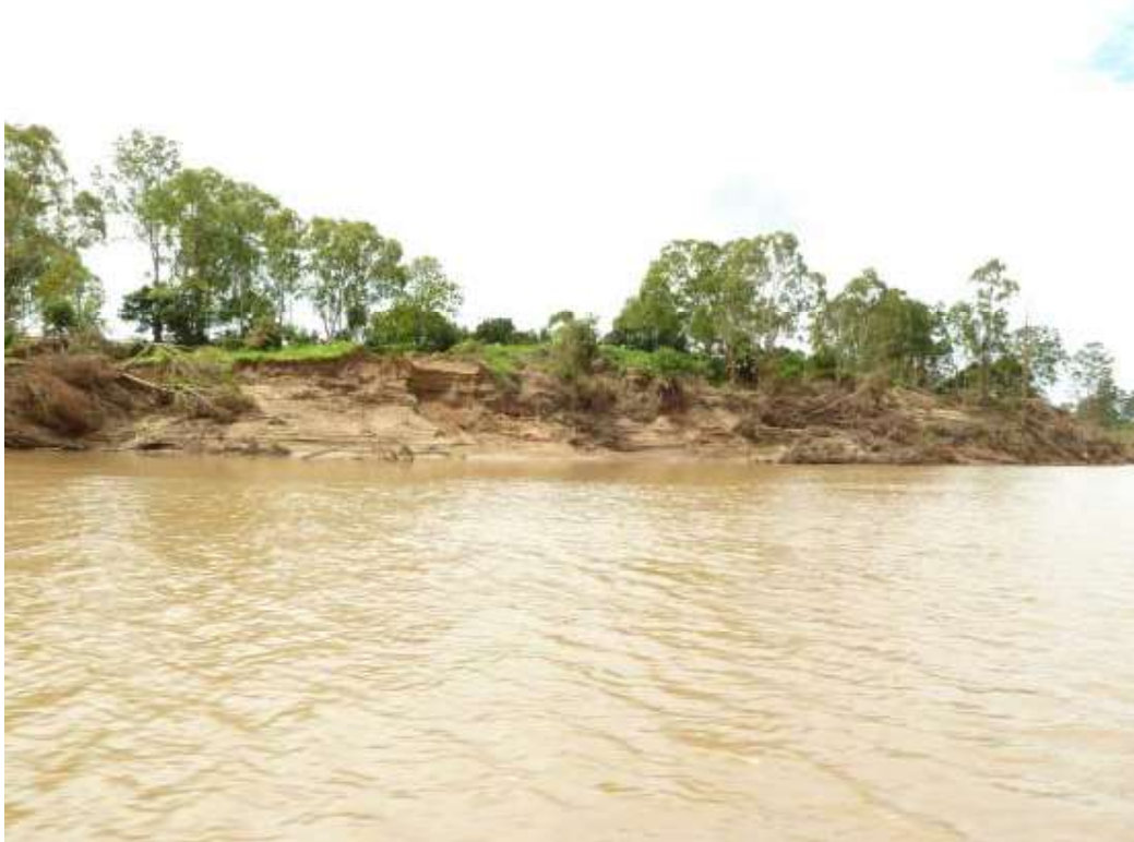
Photograph 10 River bank erosion at Moggill opposite Six Mile Creek.
