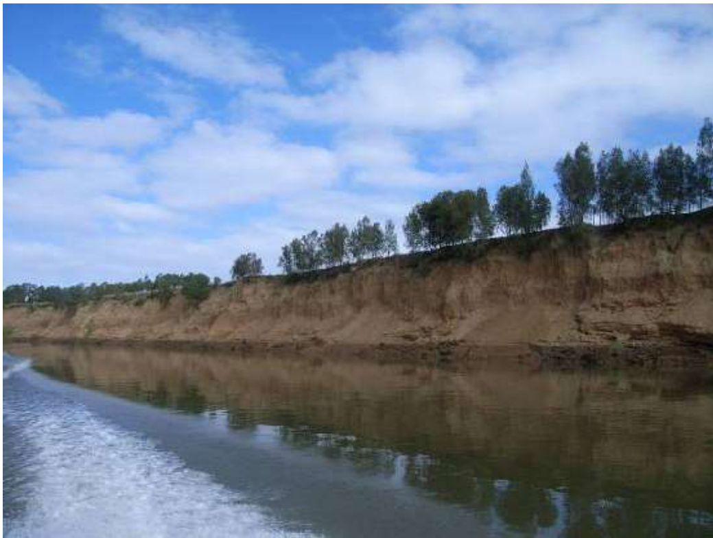
Photograph 11 Severe erosion of river bank Moggill, adjacent to Avonmore St.
