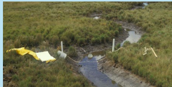
Photo 9: Smooth-sided runnel that mimics a natural channel, Coomera Island.
