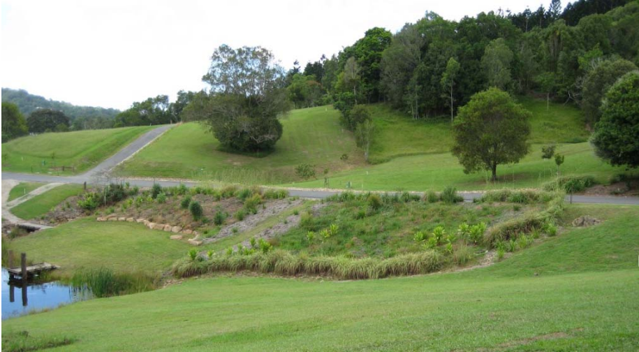
Photo 2. Vegetation used to intercept run-off from a road (Photo: Gay Deacon)
